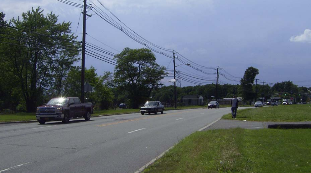
Lack of Sidewalks on Pfeiffer Boulevard
